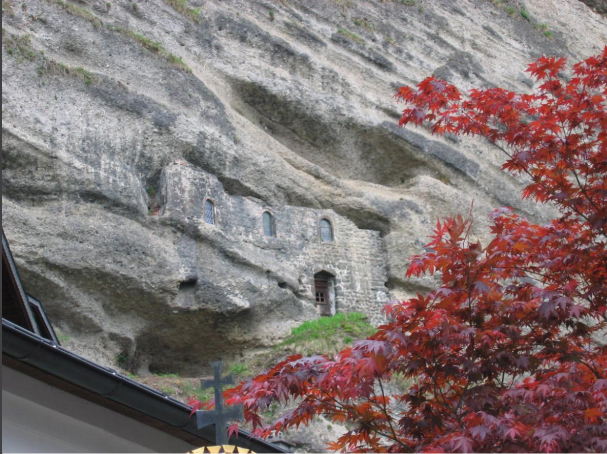
House in the stones Photo by Sr. Jayne Helmlinger, CSJ
