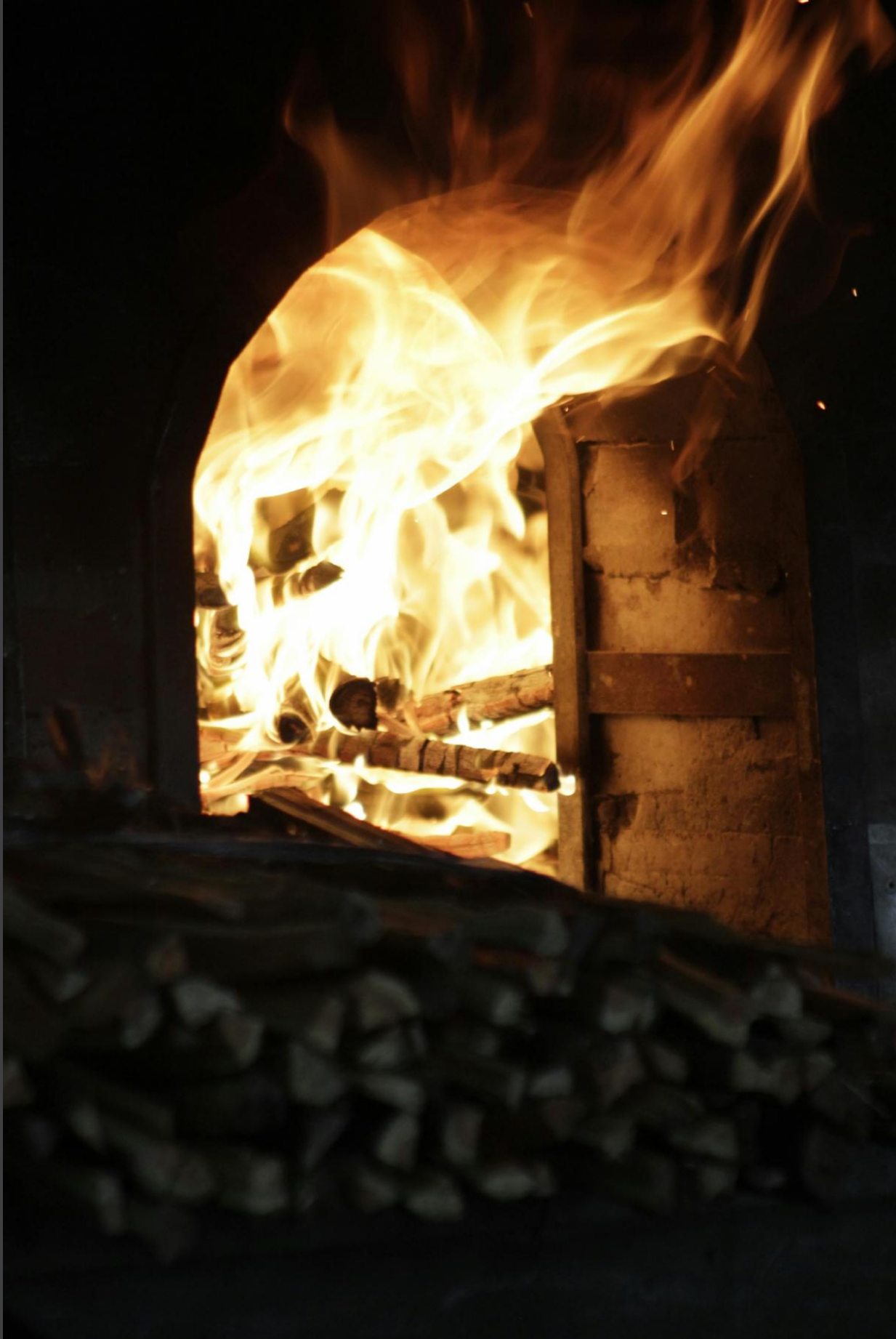
Flames in Furnace Photo by Tiago Silveira
